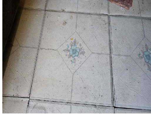
1821-2 12"x12" Floor Tile/Adhesive (x2 Layers) Interior Bathroom
