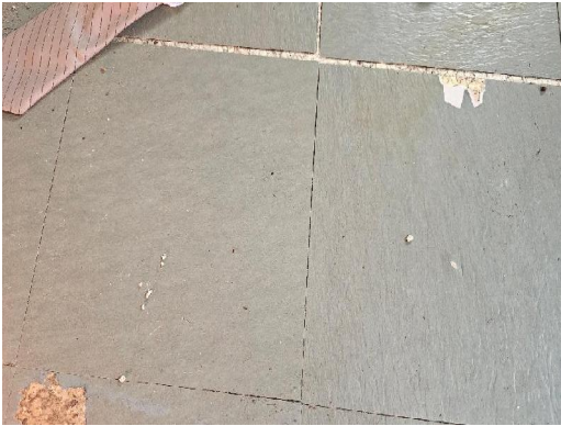
1821-3 12"x12" Floor Tile/Adhesive Interior Bedroom
