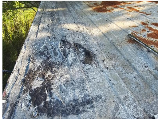
1821-4 Roof Coating/Silver (2% Chrysotile) Tar Typical Exterior Roof
