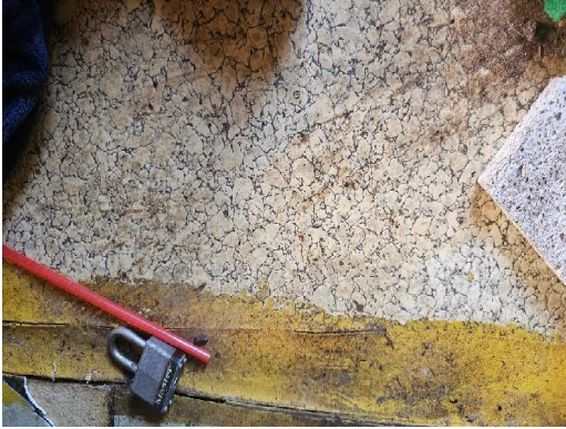
1821-1 Rolled Flooring Interior Kitchen/Hallway
